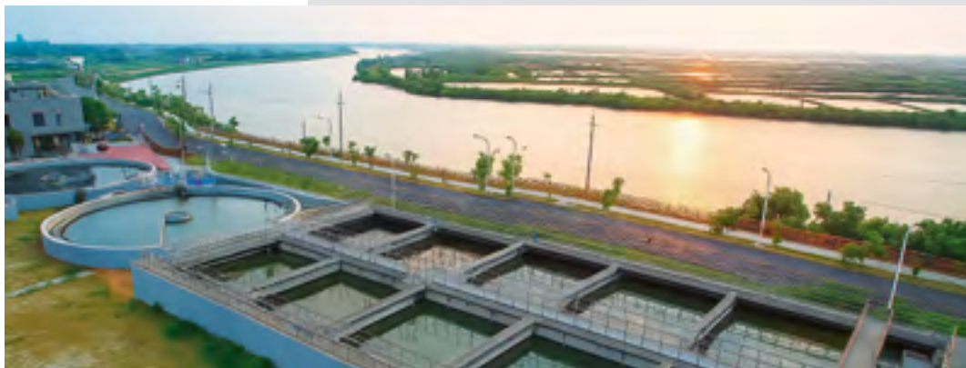
Aerial view of Annan Water Resources Centre
